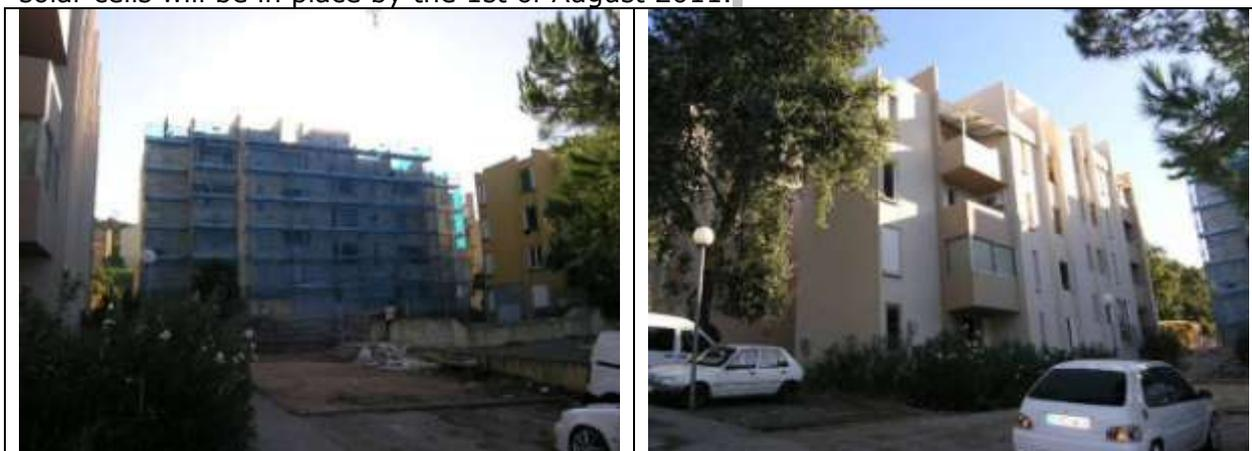
Rehabilitation work is under way although greatly delayed due to the roof surface being too weak to support solar panels. It therefore had to be reinforced and water tightness improved. There is a chance that we'll pass Crescendo's deadline for the rehabilitation work, but solar panels should be in place.
